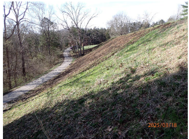
Bare soil on downstream face
