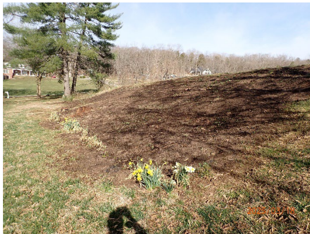
Bare soil on downstream face
