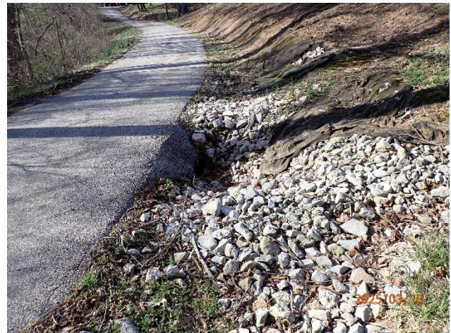
Exposed geotextile
