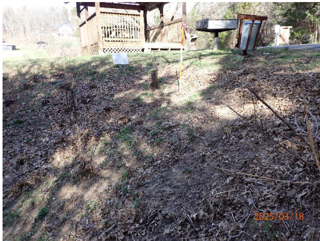
Erosion in left groin
