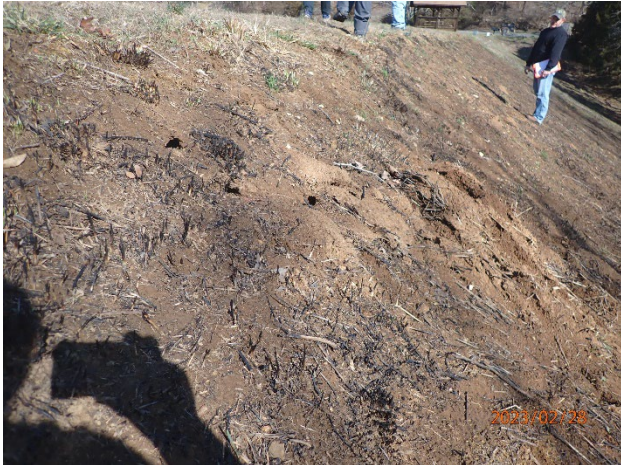
Varmint holes on downstream face
