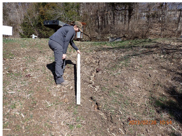
Erosion in left groin
