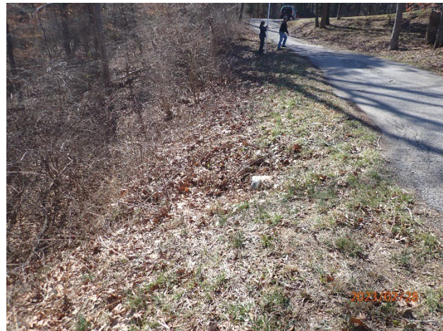
Brush and erosion at culvert drains near toe of dam
