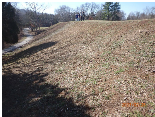
Bare earth on downstream face
